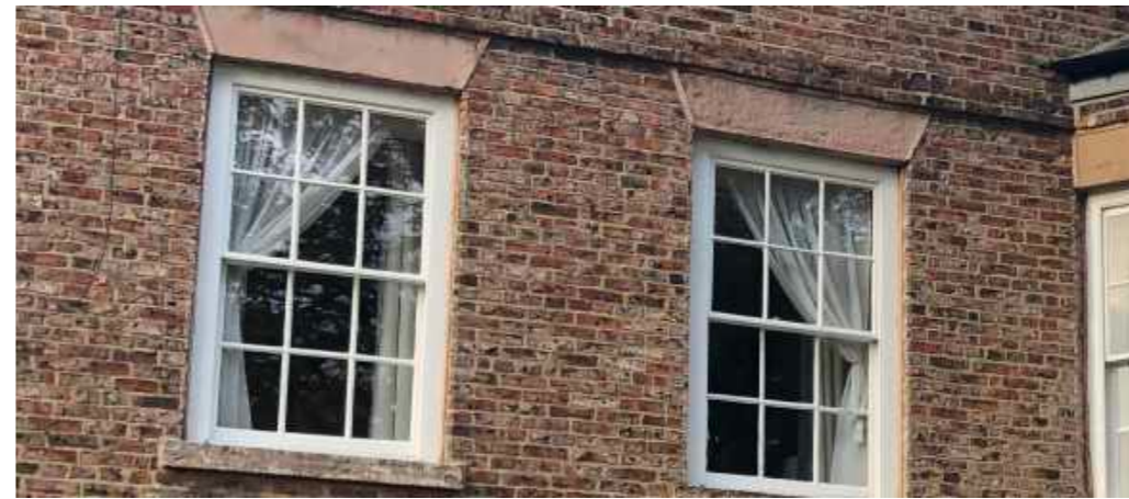
ORIGINAL SASH WINDOWS
